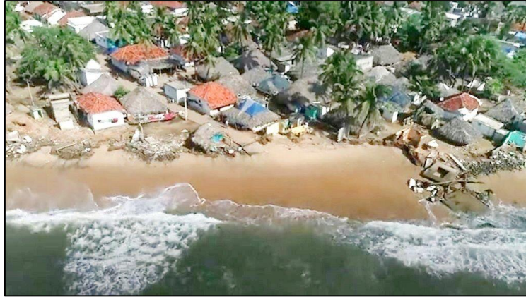
Figure 7: Shoreline erosion damaging homes and community infrastructure, illustrating the social and livelihood risks associated with climate-induced coastal change
